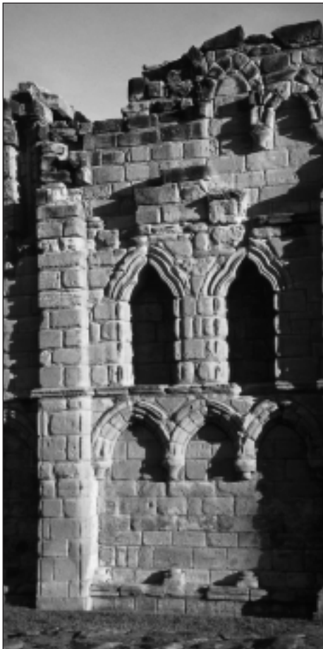
In the priory there were many uses for arches, some were structural, such as doorways, windows and vaulting. Others were decorative, such as for niches and wall decoration.
