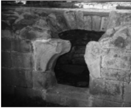
An oven in the kitchen area. It was heated to a high temperature by burning wood or coal inside, before the bread was placed inside to bake.
